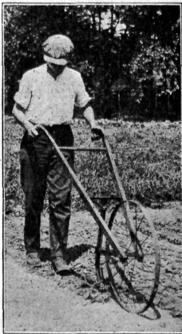
FIG. 7.—A single-wheel type of hand cultivator. Such an implement reduces considerably the labor of stirring the soil.
